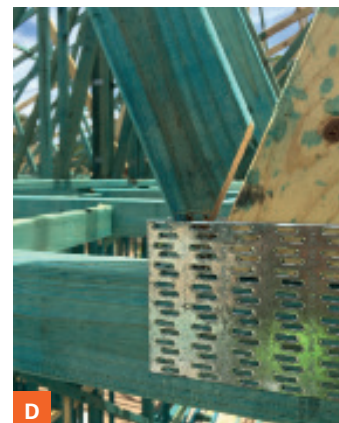
A Topchord broken out B Broken web C Nailplate dislodged D Wrong nailplate placement
