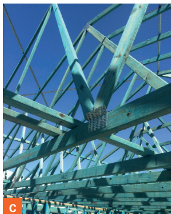
A Topchord broken out B Broken web C Nailplate dislodged D Wrong nailplate placement
