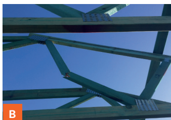
A Topchord broken out B Broken web C Nailplate dislodged D Wrong nailplate placement
